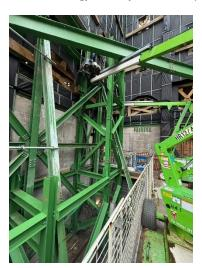
January's focus was overcoming challenging aspects of the temporary works scheme. The facade retention required sequential adaptions to coordinate and release the concrete pours of the ground floor slab and basement liner walls.
